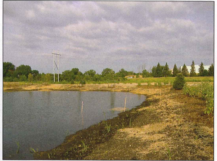
Stakes mark the different wetland zones during planting.
